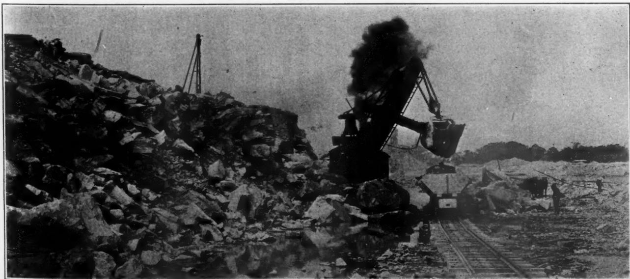
Shovel Loading Cars on Track
